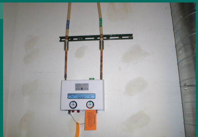
MediTrac® CMT connection to Dental Manifold.
