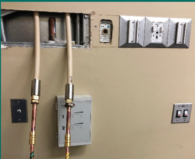
Flameless addition of medical gas outlets
