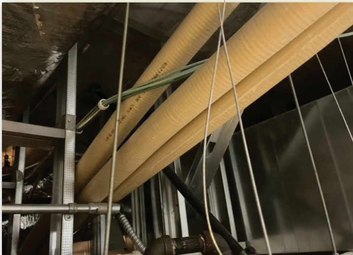
2" MediTrac CMT system above ceiling grid.
