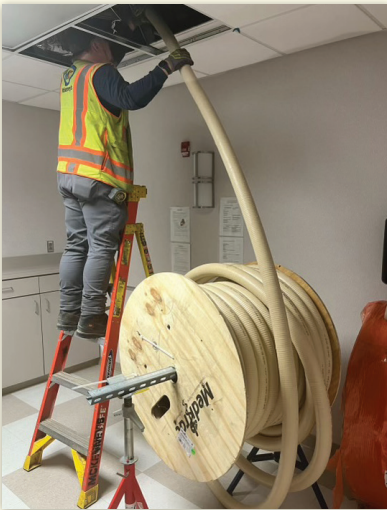
The start of multiple runs of 2" MediTrac piping.
