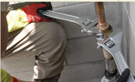
Fitting make up
