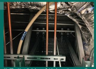
$\textit{MediTrac} {}^{\circ} \textit{installed above a finished operating room ceiling.}$
