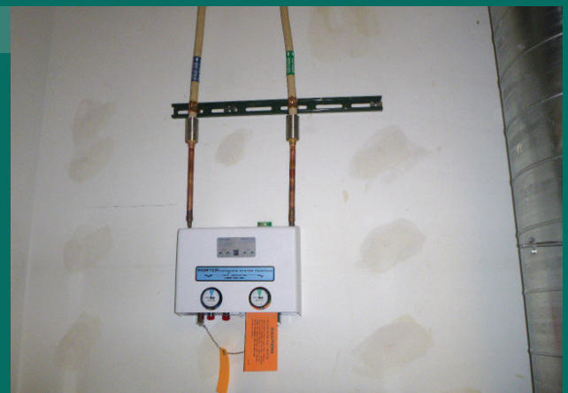
MediTrac® CMT connection to Dental Manifold.
