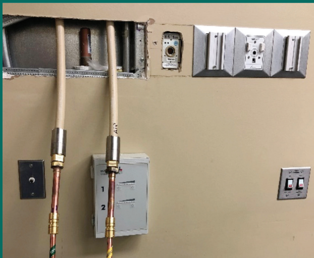
Flameless addition of medical gas outlets
