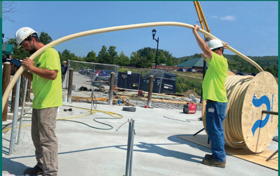
Oxygen main line for medical center.
