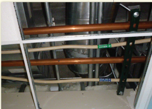
MediTrac ® installation above finished ceiling.
