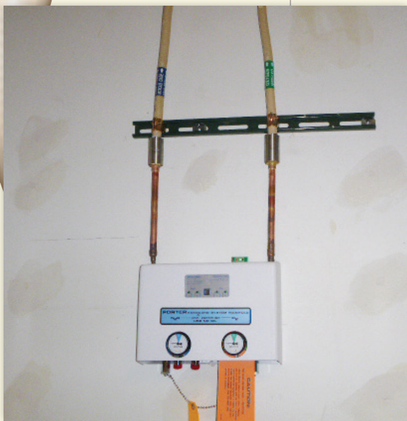
MediTrac® connection to Dental Manifold.
