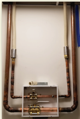
New zone valve box, with MediTrac installed for oxygen.
